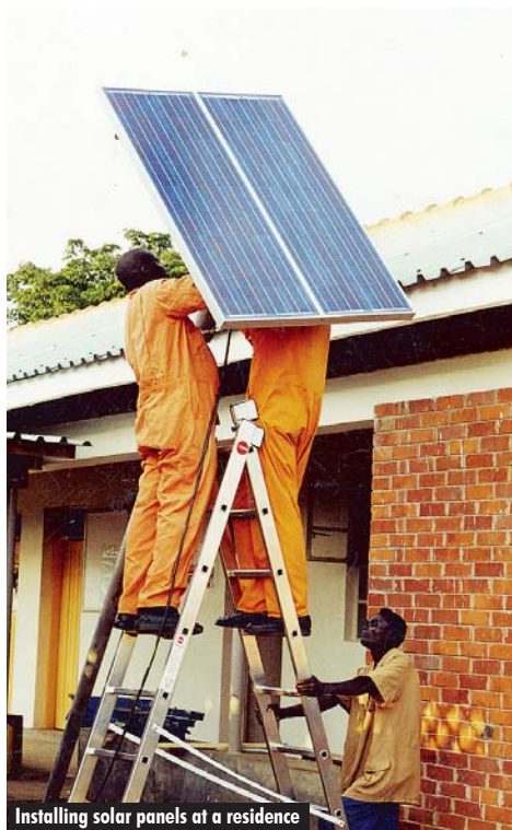
Installing solar panels at a residence
