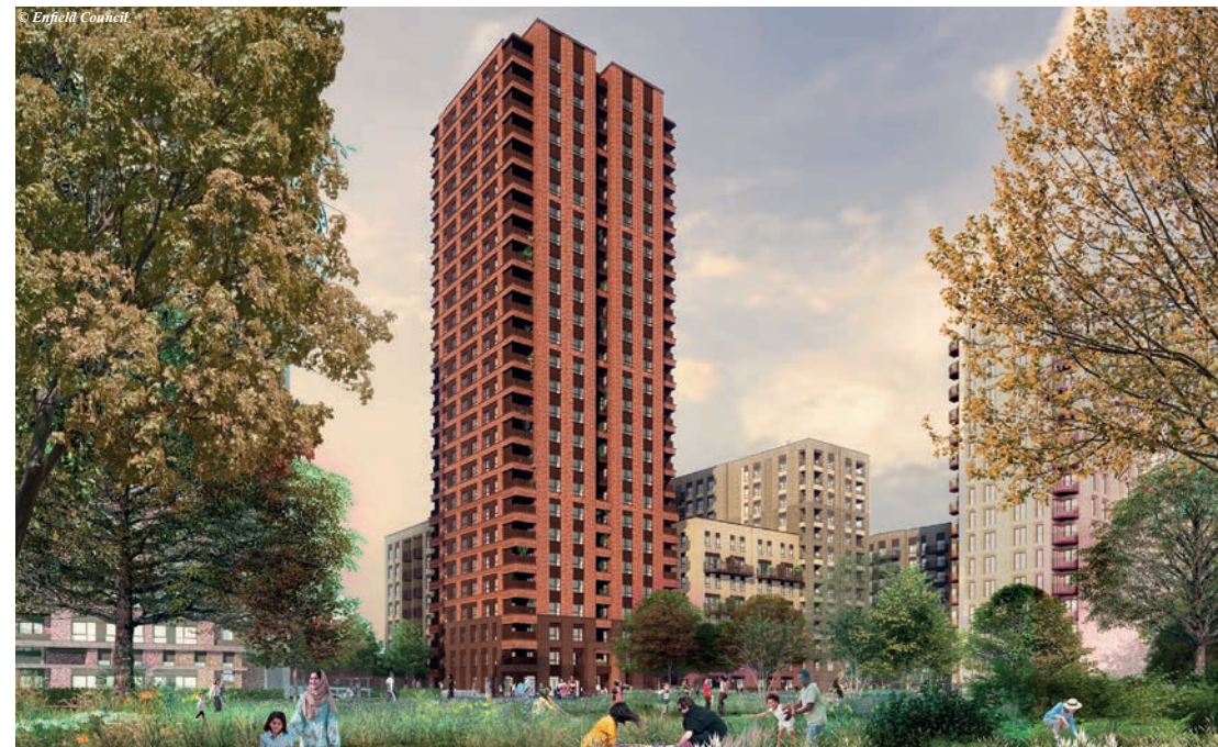
The proposed Joyce and Snells Park estate regeneration in Angel Edmonton; (top, l-r) the Meridian Water regeneration scheme has seen the first residents moving into their new homes
