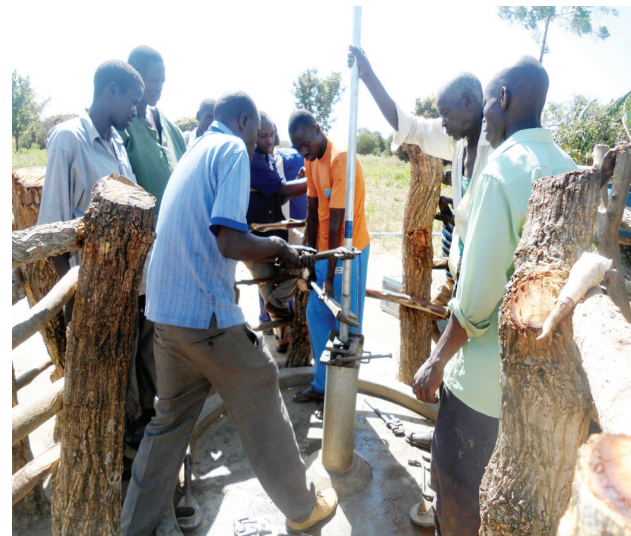
Handpump mechanics carrying out repair works
