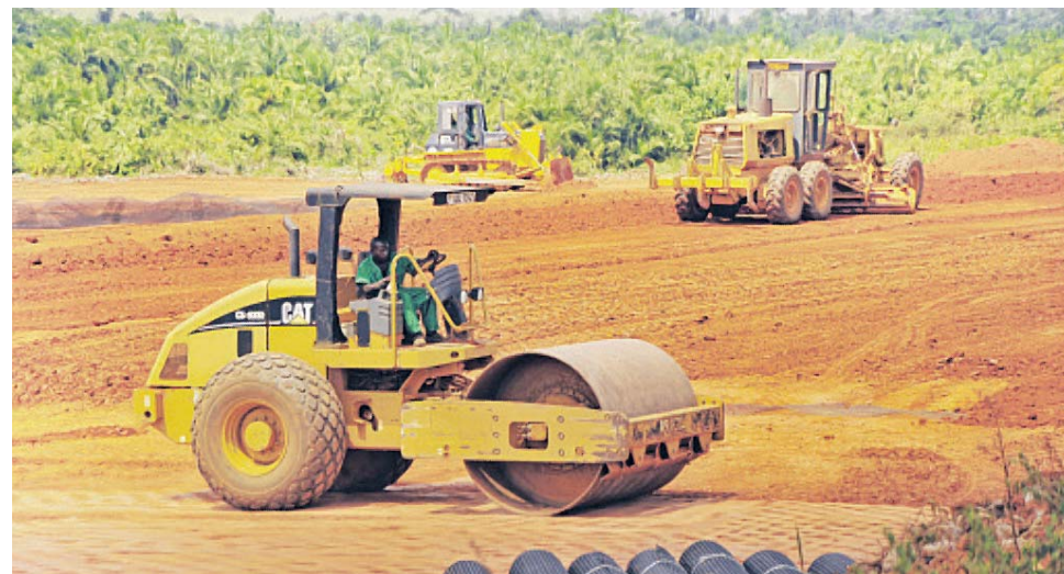
Contractors grading Kyagalanyi Coffee Processors factory site at the Uganda Industrial Park in Namanve
