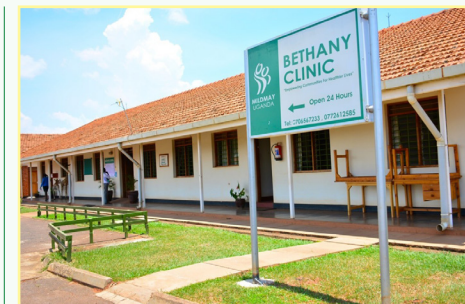
Part of the front view of Bethany Clinic
