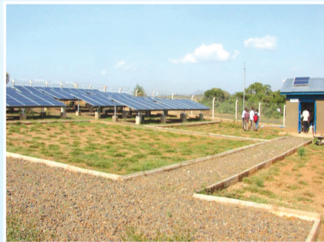
Solar panels used as energy for pumping water
