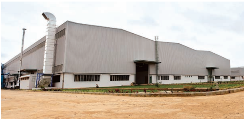
All sources of pollution are equipped with suitable pollution control equipment
