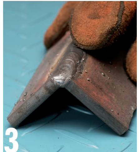
3 An external corner fillet is where the two sections meet at the corner forming a 90-degree edge prep. This leaves a rounded, neat corner requiring little to no dressing with the grinder. Additional beads can be run on the inside for increased joint strength.
