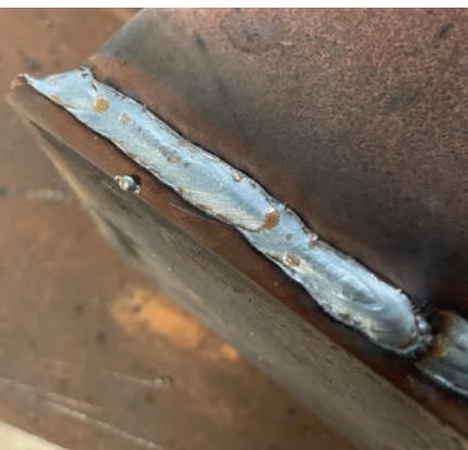
5 A lap fillet can sometimes be used in place of a simple butt joint, providing the design allows for the misalignment. The benefit of the lap fillet over the butt joint is it requires little preparation and can be welded on both exposed edges, giving greater strength.
