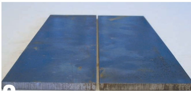
For thicker butt joints over 3mm but less than 5mm, use an open butt arrangement. The gap should equal half the plate thickness. Note that the welding process will also influence joint preparation. The more welding current available, the easier it is to achieve penetration. If you are welding with limited current on a small machine, err on the side of more preparation than less.
