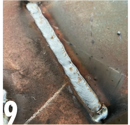
9 Another benefit of using the correct weld preparation is that sufficient joint strength can be achieved without excessive reinforcement, or convex weld bead. This creates a neater joint and requires little dressing with a grinder to achieve a clean surface.
