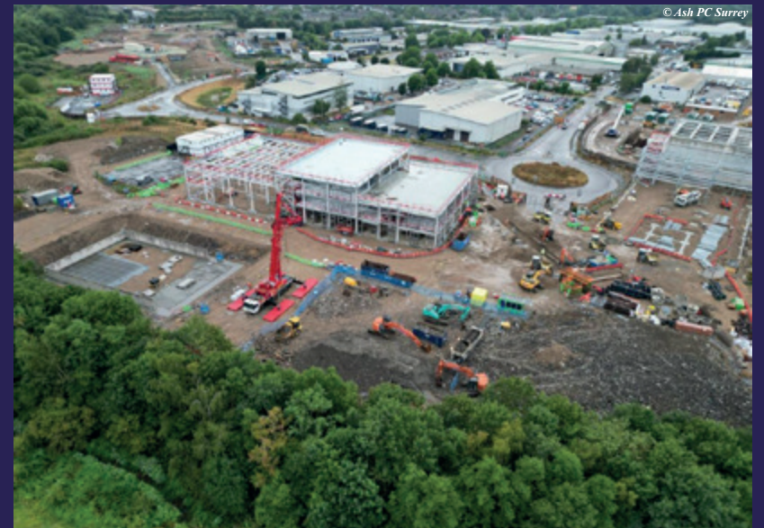
Aerial view of the new Guildford Borough Council depot under construction
