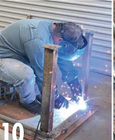
With the legs square they can now be fully welded in place. Place a couple of strategic tack welds on each corner of the legs where they come up against the table top and the base frame. Now weld the legs to the base frame (shown), and also on the inside to the tabletop.
