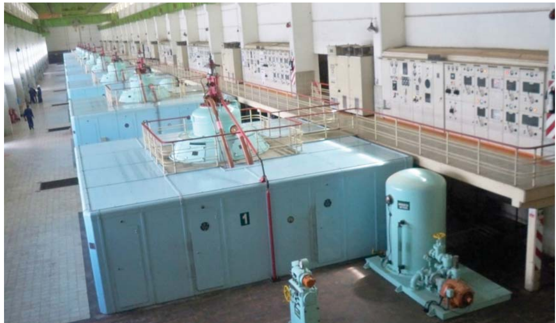
Nalubaale power station generators. The station has a generation capacity of 180MW. It supplies power to Jinja town and the surrounding areas
