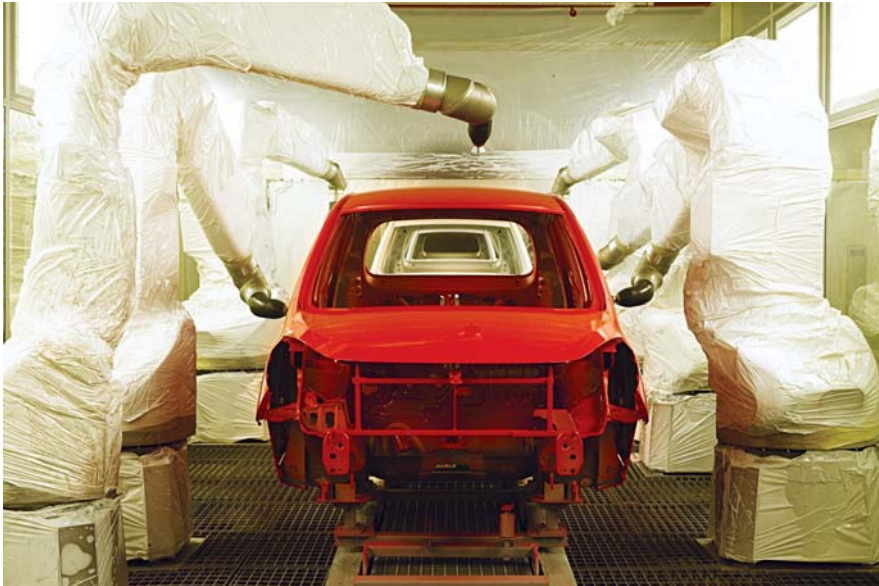
The paint shop which is 60 percent automated, is fitted with the latest equipment, and uses environment friendly water based process and robotic paint application.
