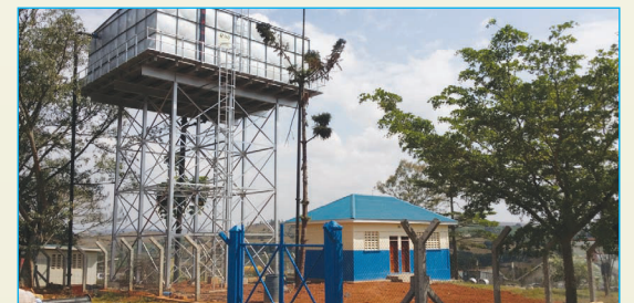
Photo 10: Completed 200m³ reservoir tank and chlorine house at Muko hill in Ntungamo town
