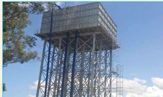
Photo 4: Constructed 340m³ steel water tank in Mayuge Town
