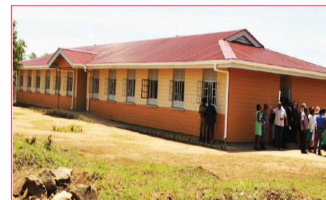
A Girl's dormitory at Nakapiripirit Primary School constructed under the Irish funded KPEP
