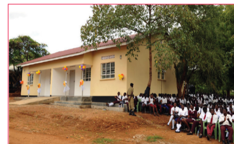
Twin Staff House constructed by the Ministry of Karamoja Affairs at Moroto High School
