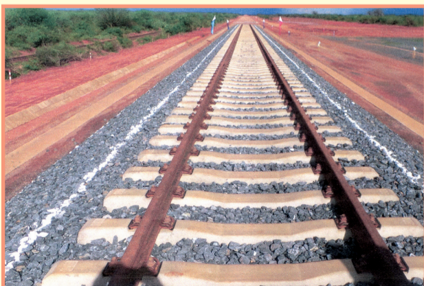
The Standard Gauge Railway tracks
