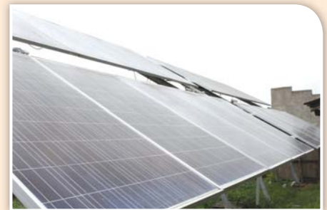
5kw solar micro-grid providing electricity to 120 Households in a fishing village, Kasese
