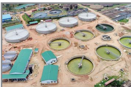
The substantially complete Bugolobi-Nakivubo waste treatment plant will treat 45 million litres of waste water every day.
