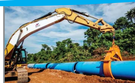
Katosi Project: On going pipe laying pipe
